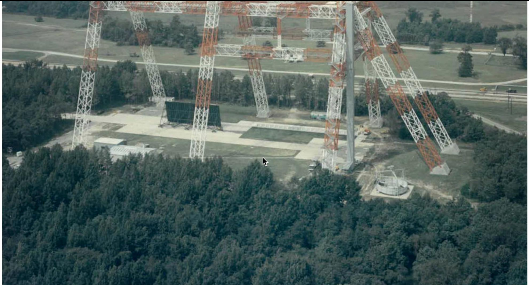
Pictured is Langley's 250-foot high Lunar Landing Research Facility. Apollo astronauts perfected their piloting and moon walking techniques here with a simulated lunar surface. The site was named a National Historic Landmark for its contributions to manned space flight programs.
